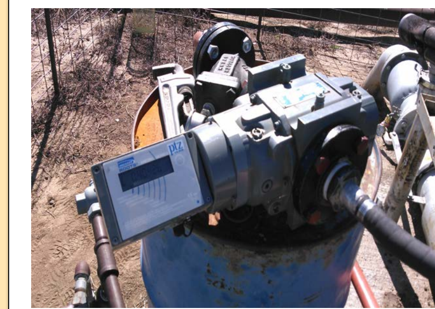
Natural gas meter: Measures the flow rate of the gas into the engine
